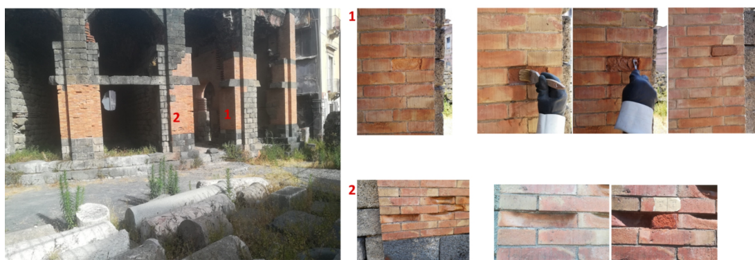
Fig. 1 - Case study: Odéon of Catania - steps of applications of geopolymeric mortars.
