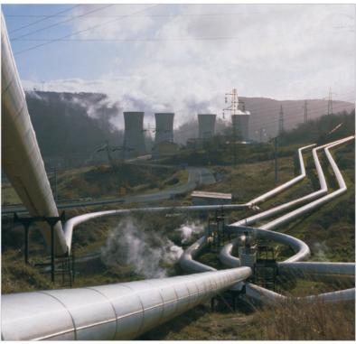
Larderello: steampipes of the geothermal power plant (courtesy of ENEL SpA)
