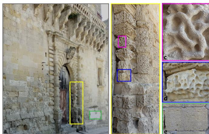
Fig. 4 - a) Degradation of the Calcarenite di Gravina on Palazzo Santoro, Matera; b), c), d) detail of the fossil traces deriving from the bioturbation after weathering activity (differential erosion).
