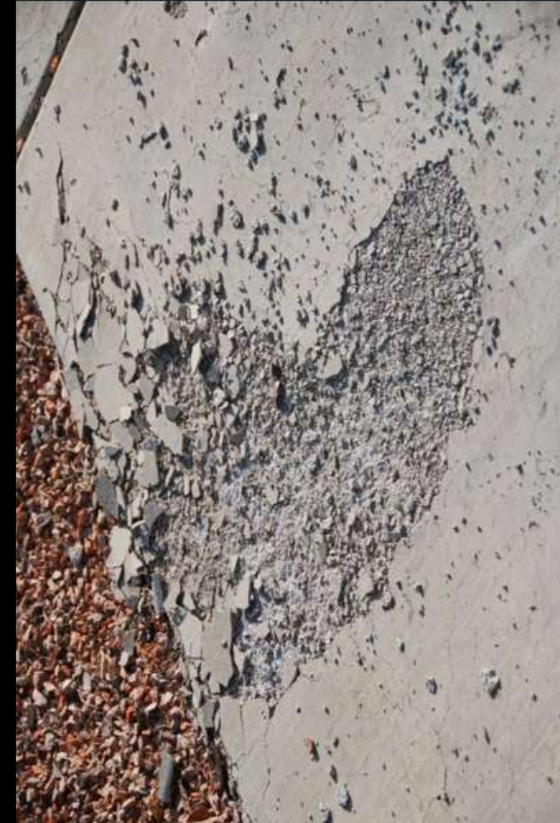
Freeze-thaw degradation
